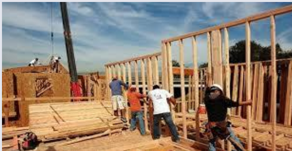
Home Remodel Construction Workers
